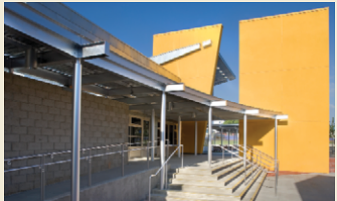
CANOPY IN FRONT OF THE MULTIPURPOSE/KITCHEN BUILDING
