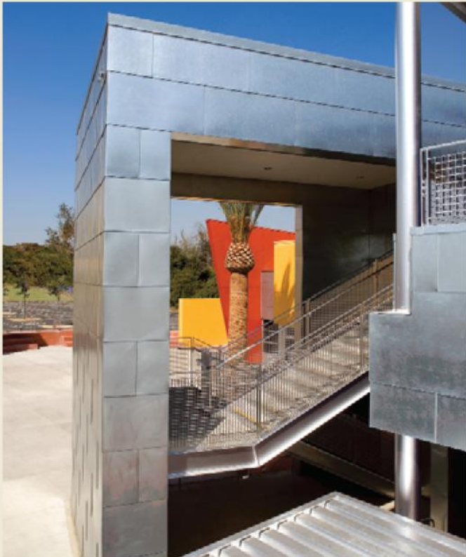
GALVANIZED METAL STAIRWELL
