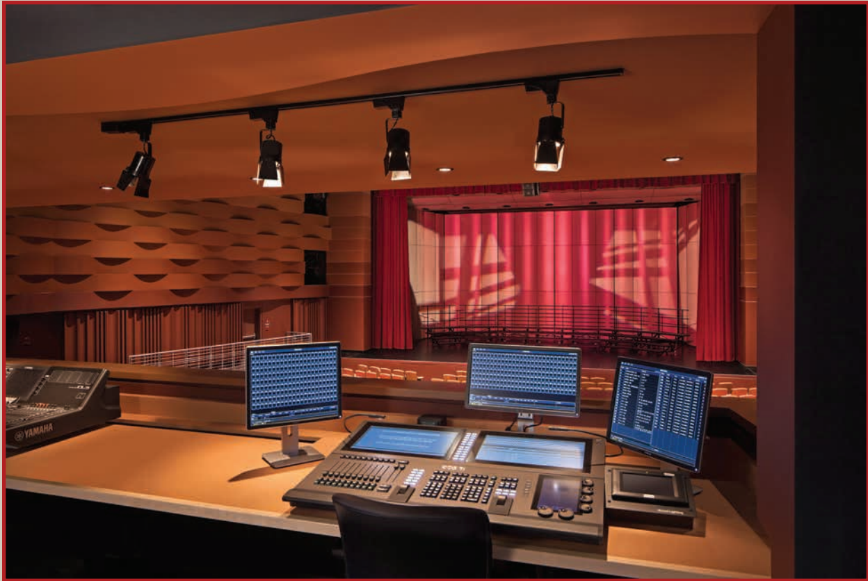
The view from the booth, showing the ETC Eos Ti lighting console.
