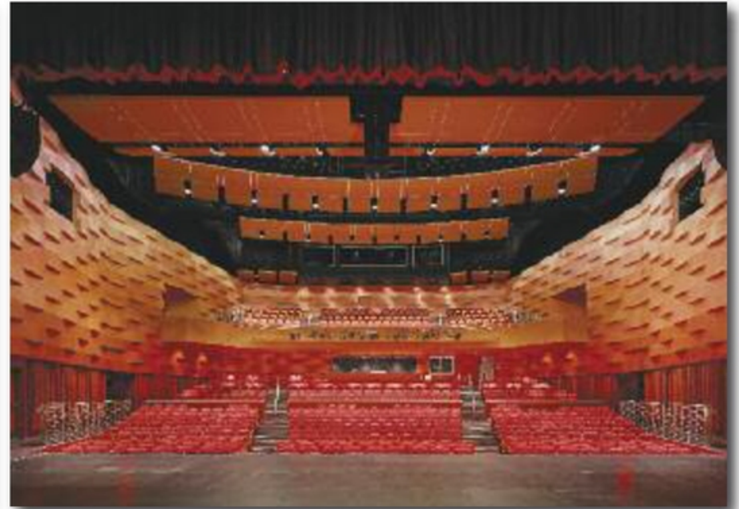
The design team worked very closely with acoustical engineers to create a system called variable acoustics, a basket weave—design shape customized to enhance reverberation time.
